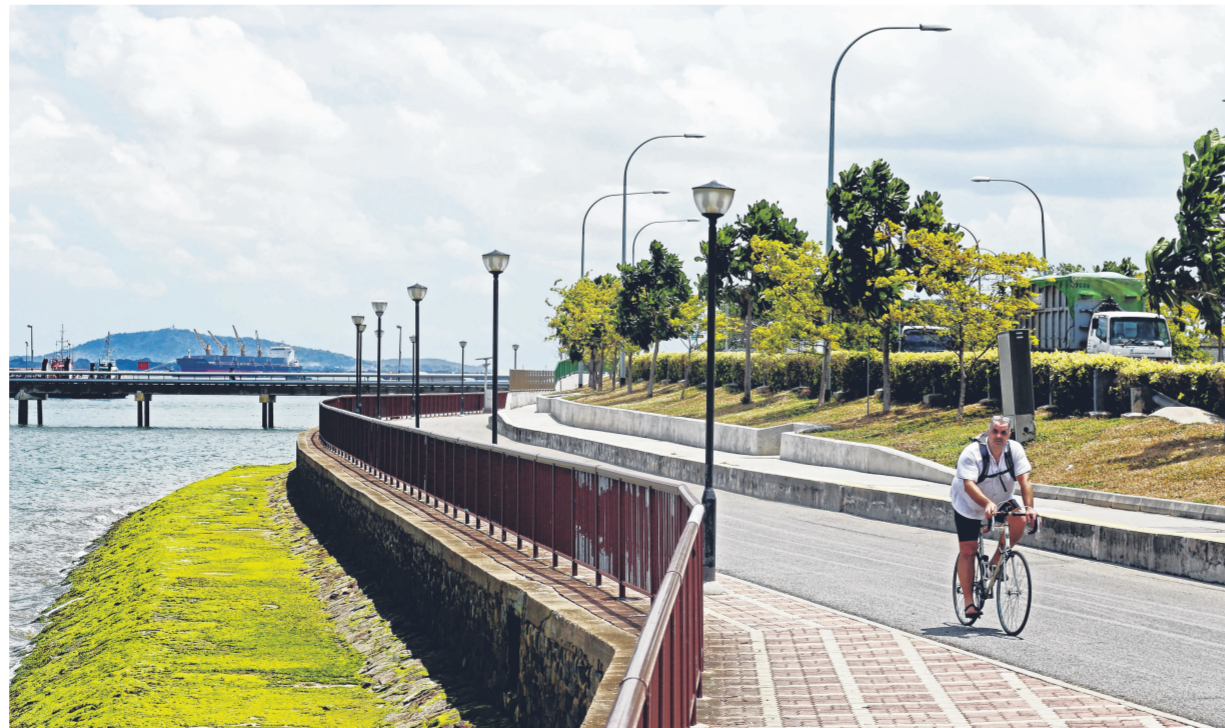
Roads like Nicoll Drive were raised to reduce the impact of flooding as sea levels rise. Prime Minister Lee Hsien Loong has said around $100 billion may be needed to protect Singapore against rising sea levels. PHOTO: LIANHE ZAOBAO
