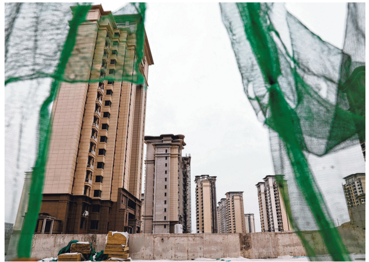
Unfinished residential buildings by China Evergrande Group. Evergrande defaulted on its bonds and was ordered to liquidate this year. PHOTO: REUTERS
